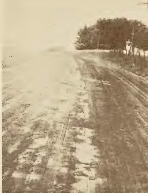
FIGURE 7.—APPEARANCE OF SURFACE AFTER FIRST APPLICATION OF OIL. NONUNIFORM PENETRATION HAS OCCURRED BECAUSE OF LOOSE MATERIAL ON THE SURFACE. THE PRESENCE OF UNABSORBED OIL ON THE SURFACE IS INDICATED BY THE LIGHT SPOTS
